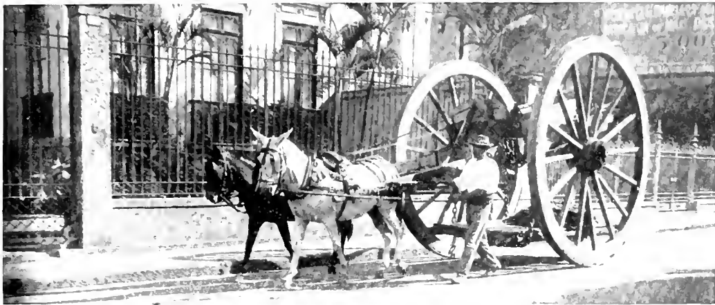
Carrying heavy goods under instead of above the axle.
